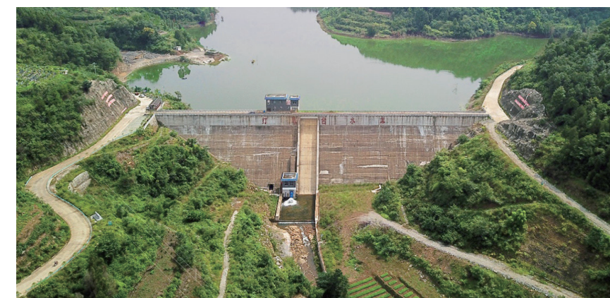
The Dagutai RFC gravity dam in Guizhou Province has a maximum height of 41m.
