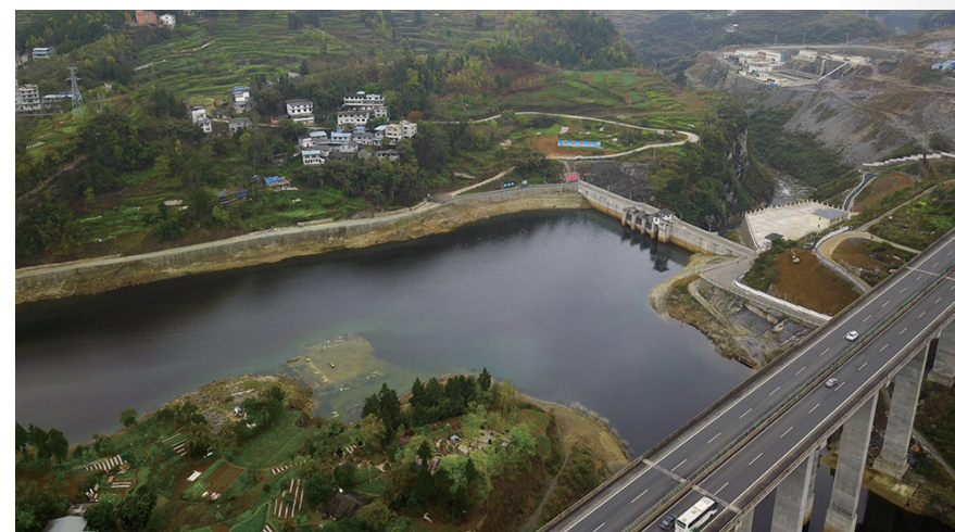
The Maoxigou RFC gravity dam in Guizhou Province has a maximum height of 44.5m.
