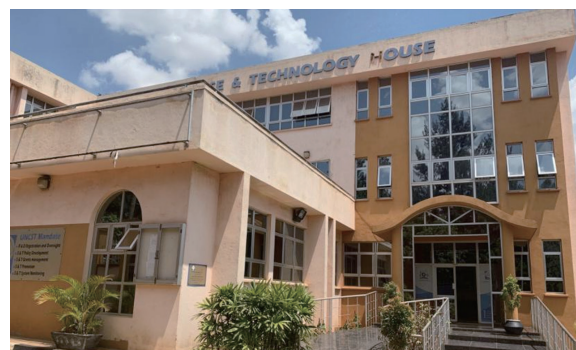
The Owner's Office in Kampala
